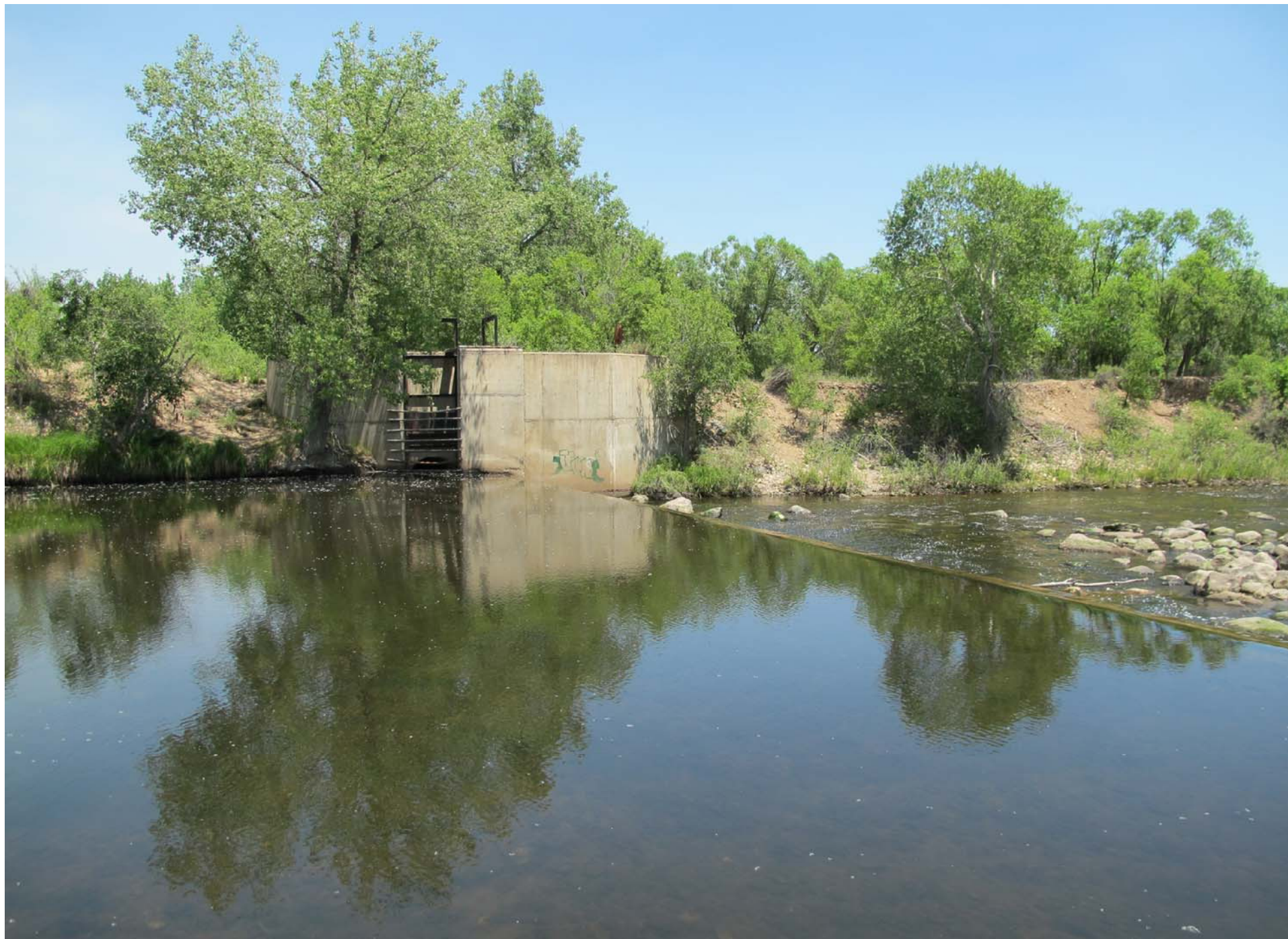
SITE PHOTO 1 VIEW LOOKING AT STRUCTURE
