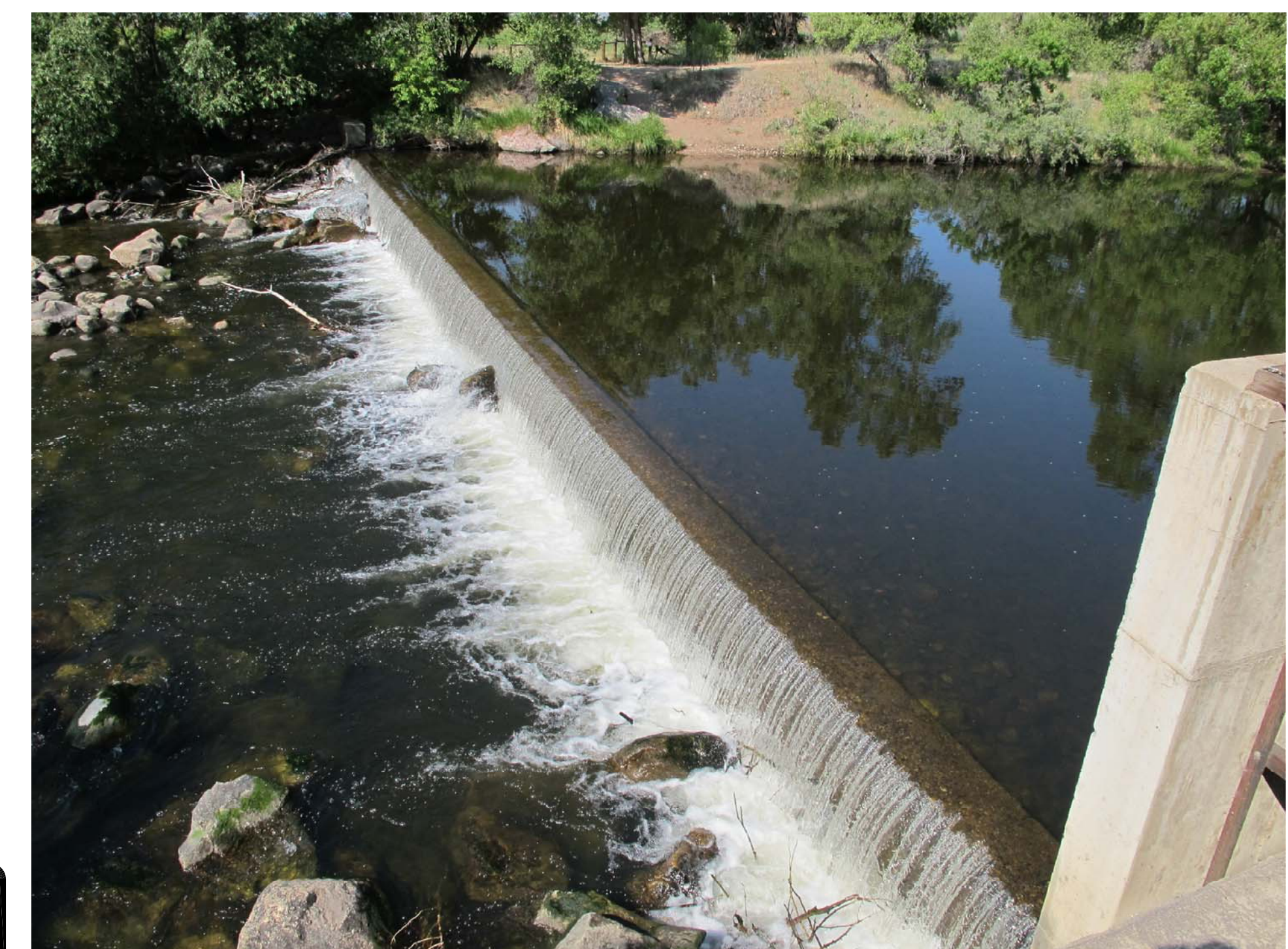
SITE PHOTO 1 VIEW FROM STRUCTURE
